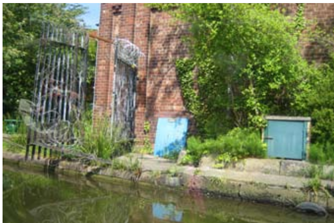
No access along eastern side of canal
