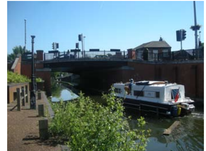
Above, the canal has a multi-functional green infrastructure role.
