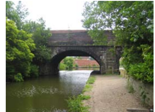
The north side of railway crossing the canal
