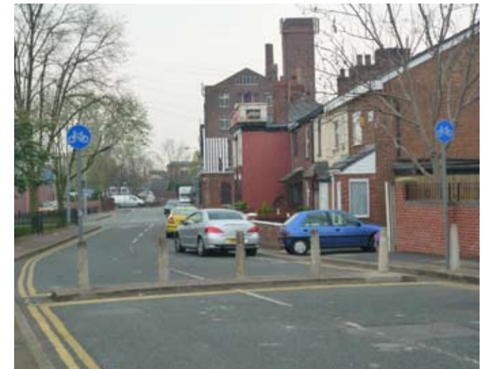
Bollard barrier between New Street and Chapel Street
