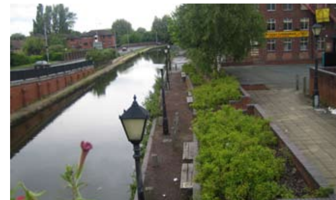
Former public realm improvement in poor condition
