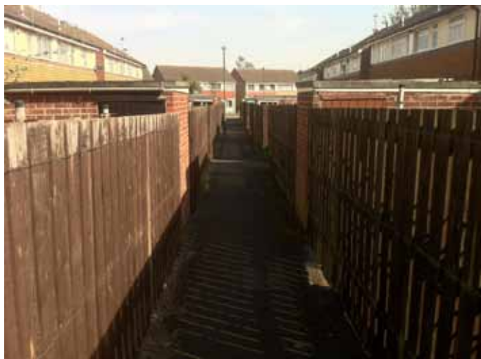
The Cross Wall flats which have recently been demolished on the site. A dark footpath leads into the properties, which feels unsafe. It also means residents are unable to park at the front of their properties.
