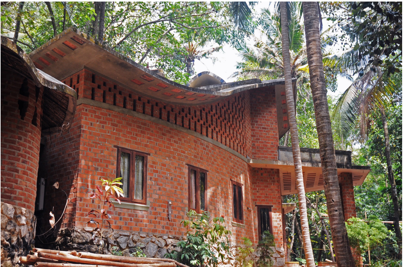
Fig. 2.3. Laurie Baker Centre for Habitat Studies, Thiruvananthapuram, Kerala
