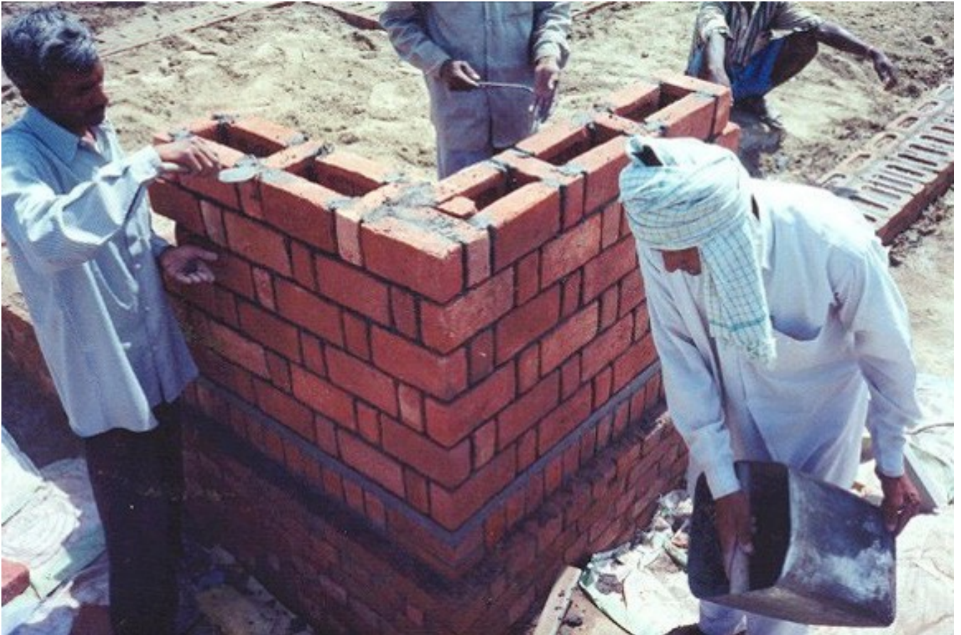
Fig. 3.10. Construction of a rat-trap bond wall
