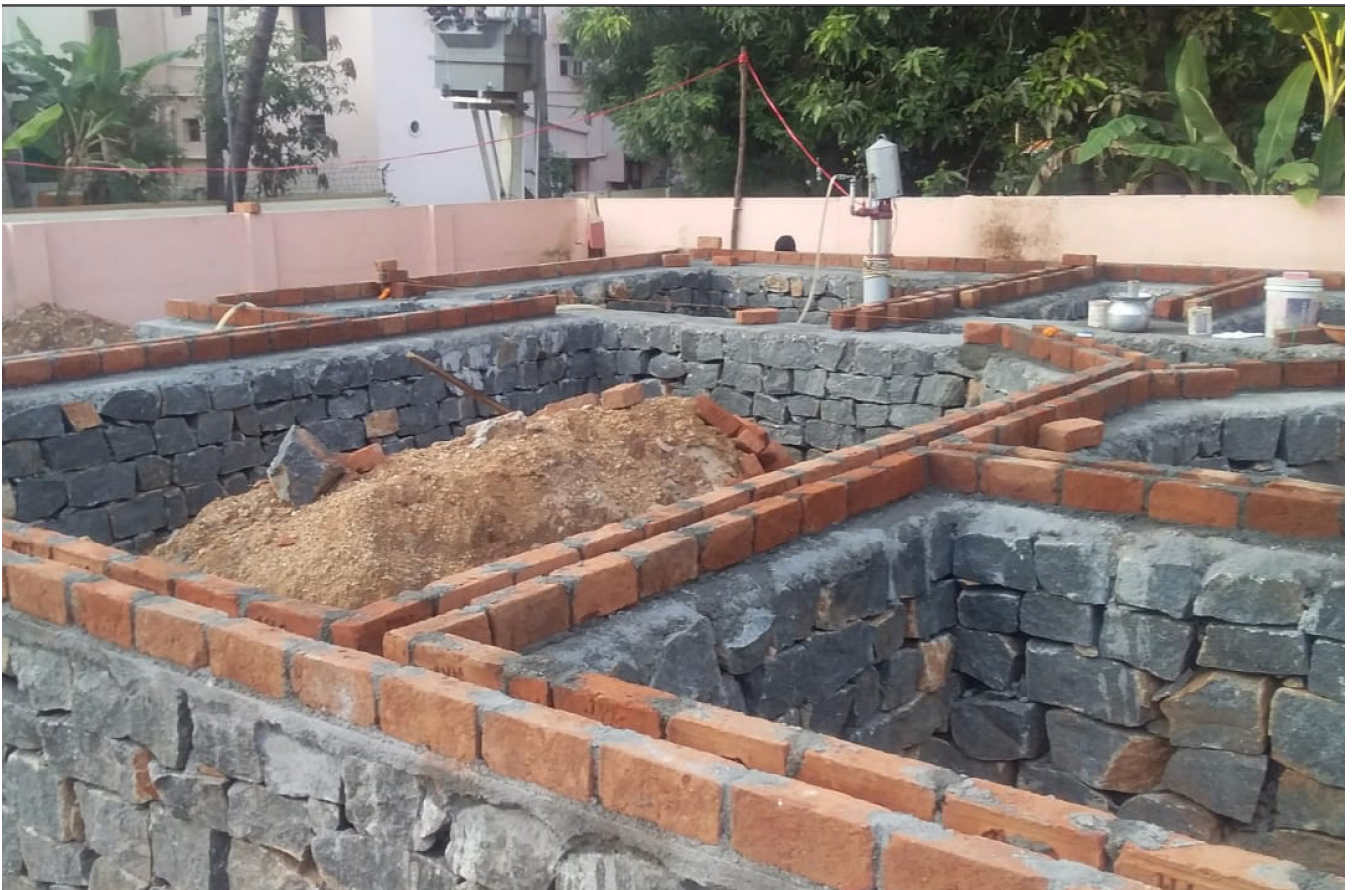
Fig. 3.11. Random rubble masonry for foundation & plinth
