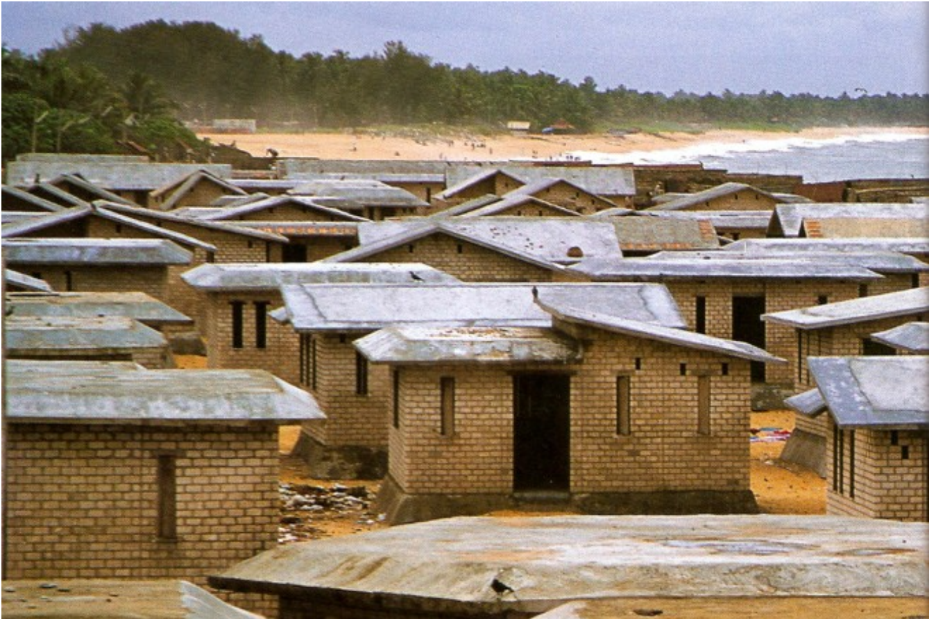
Fig. 2.14. Thangassery Housing, Kollam, Kerala
