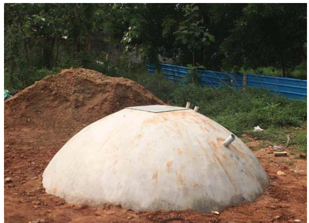
Fig. 3.6. Construction of a bio-digester
