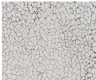
Broken tile flooring
