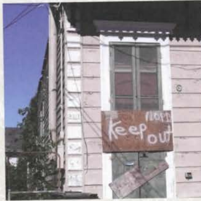
Many properties throughout the city remain boarded up.
